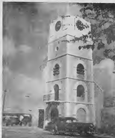
One of the early historic landmarks of Aruba is Fort Willem III on Zoutman Street in Oranjestad. The reign of King Willem III was noted for the abolishment of slavery, and the Fort was built in his honor. It serves as a clock by day and a beacon for ships by night.
